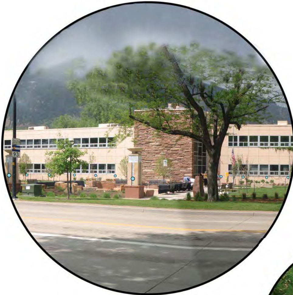
Boulder Municipal Center
