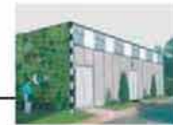
roaches run pump station
