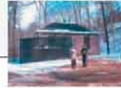
windy run pump station
