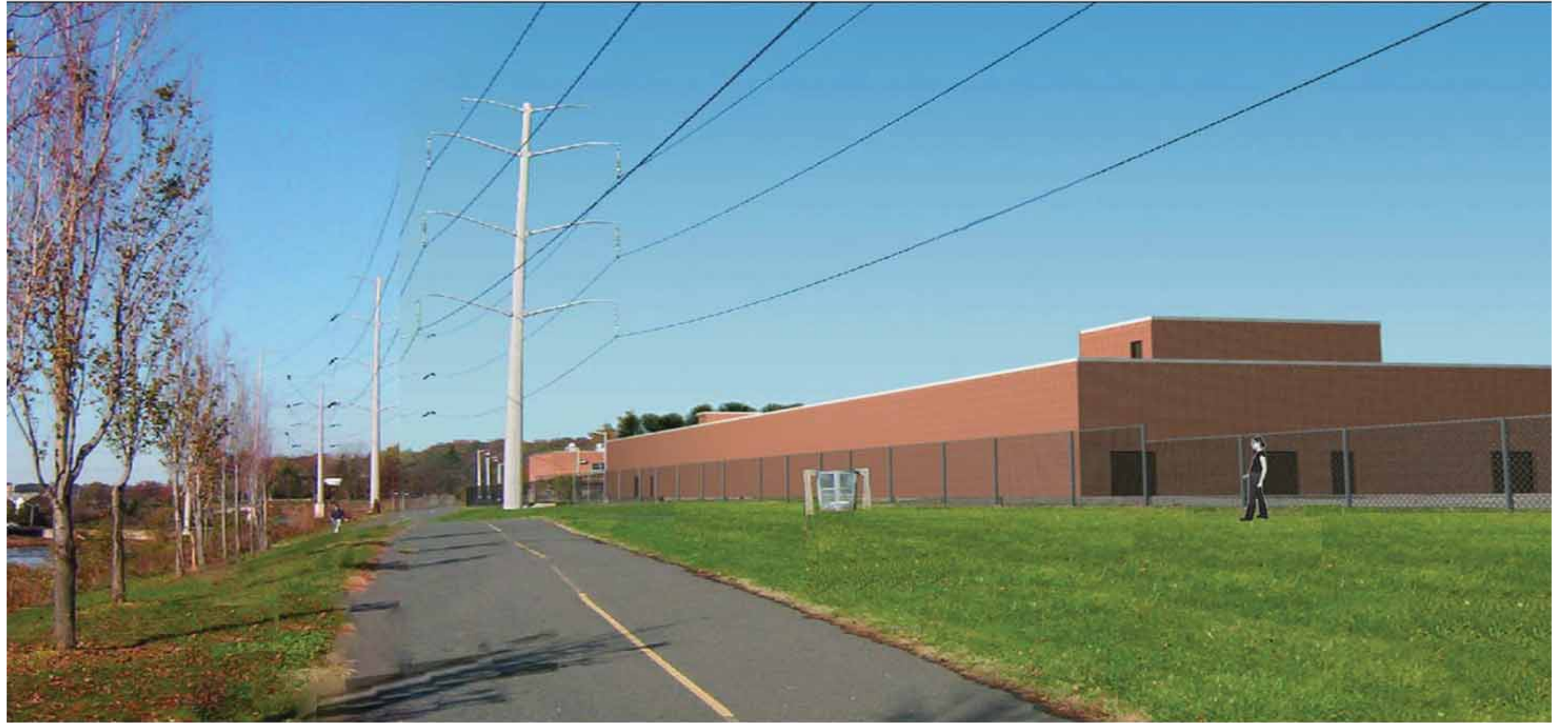
new filtration building, bike path, and river edge BEFORE
