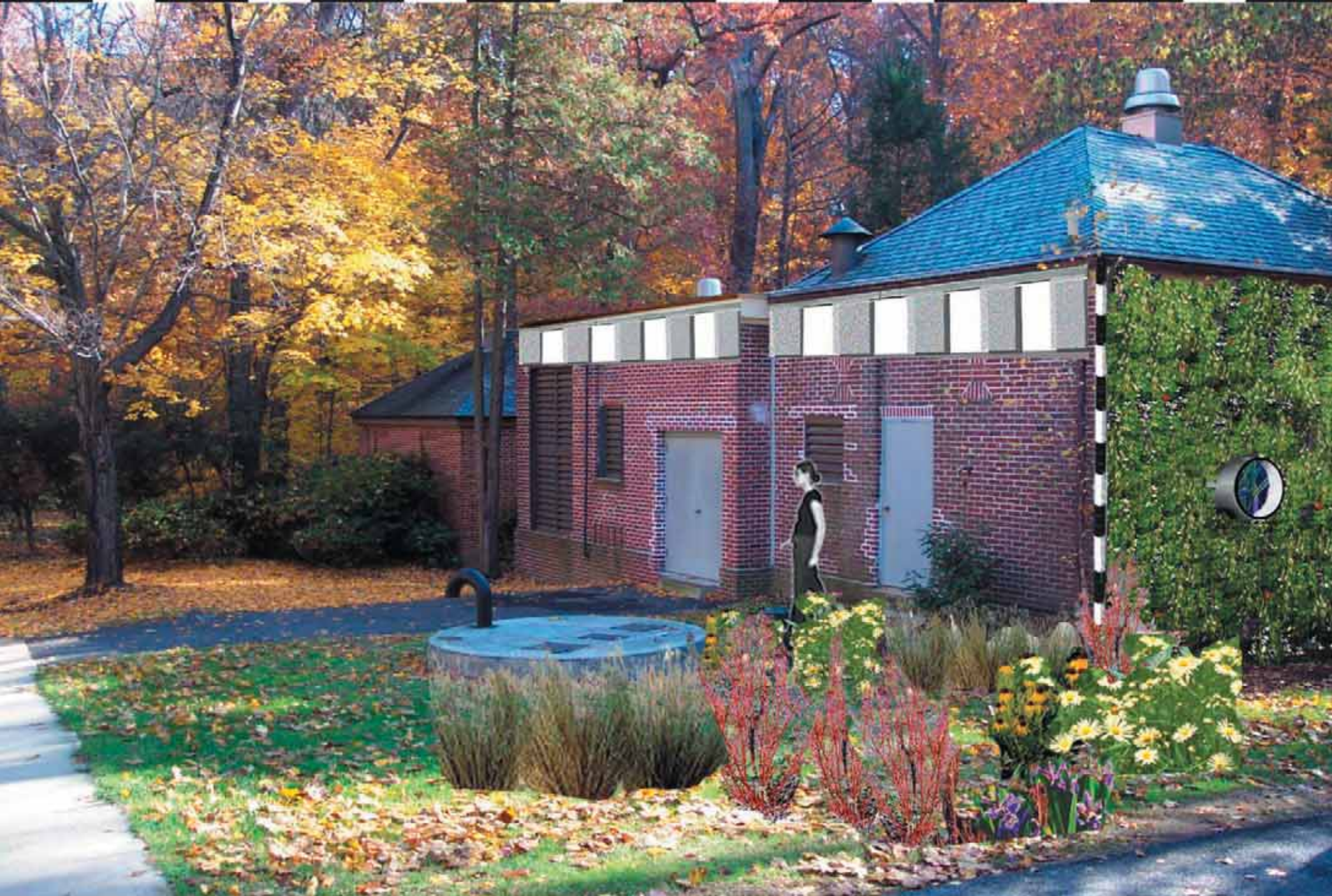
PUMP STATION WITH PLANT SCREEN, RAIN GARDEN, AND FACADE OPENING
