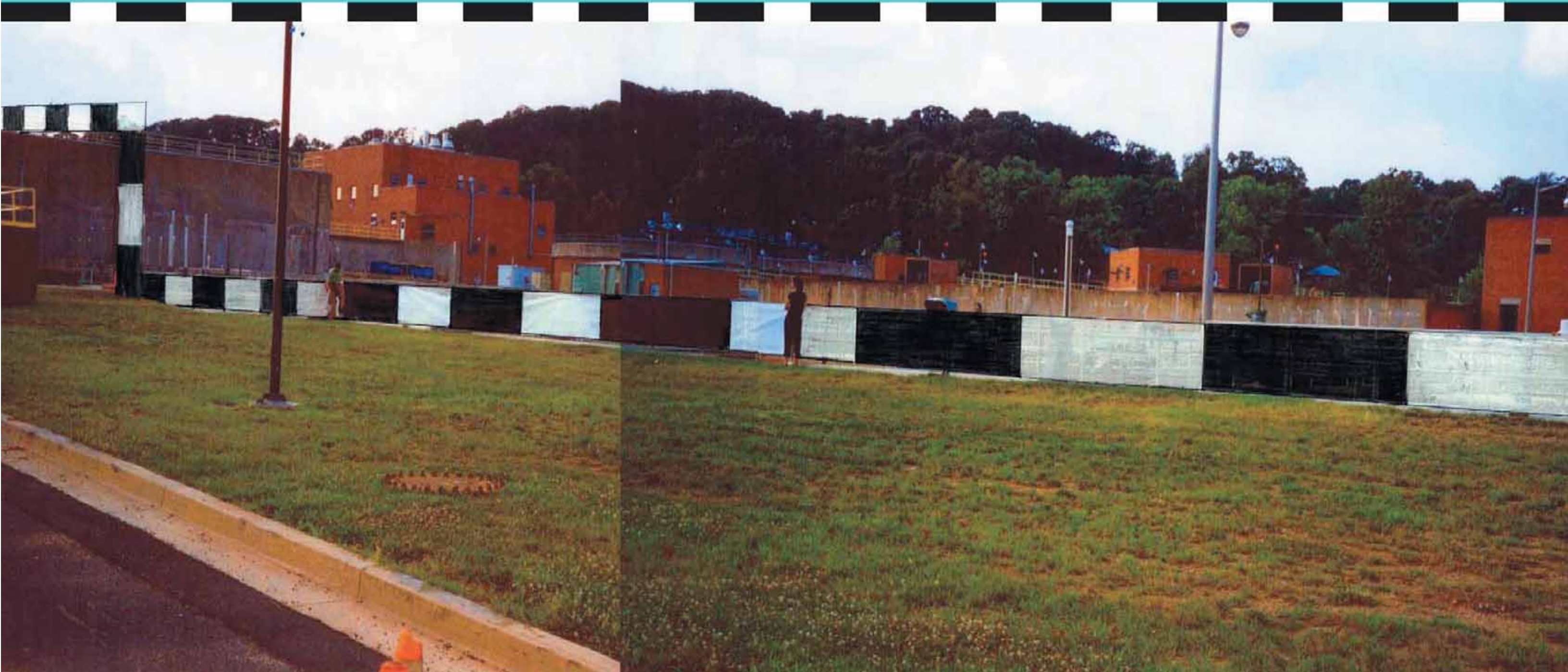
BANDED PIPE RUNNING ALONG SOUTH SIDE OF ACWPCP IN FRONT OF AERATION TANKS
