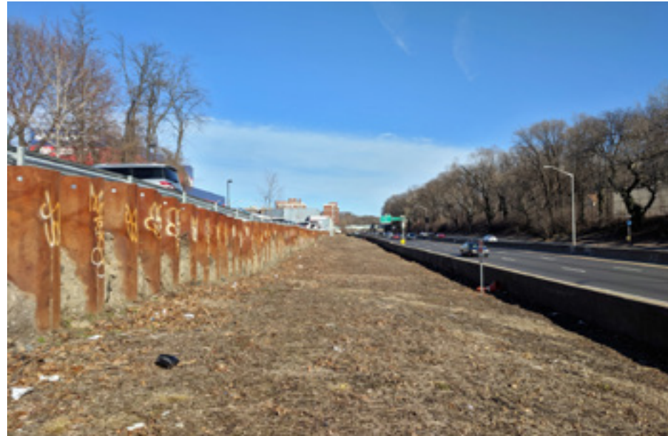
Former location of CSX railway tracks adjacent to the the Major Deegan Expressway.
