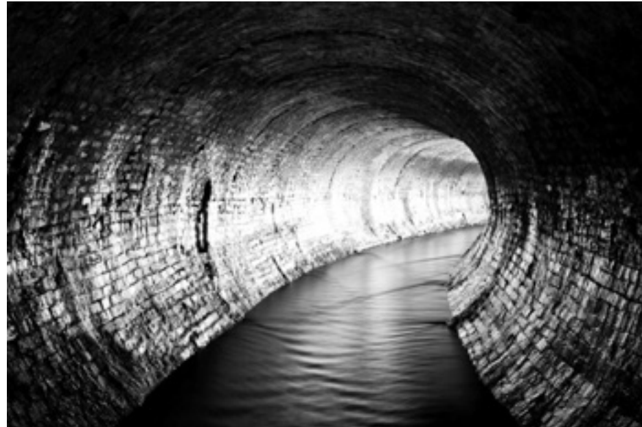
Inside the Broadway sewer.
