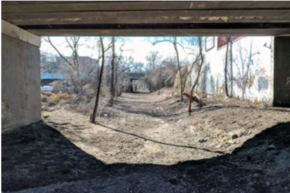
Underneath a bridge crossing the CSX corridor.
