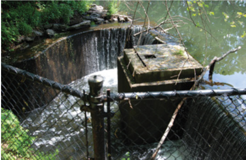
Outflow of Tibbetts Brook from the Van Cortlandt Lake into the Broadway Sewer.
